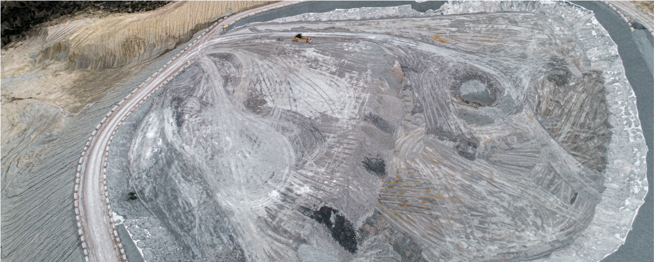
→ Cosentino®'s waste management plant
